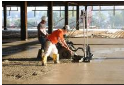
The Somero Mini Screed C is lightweight for on-deck use and equipped for many commercial applications, such as over rebar or post tension.
