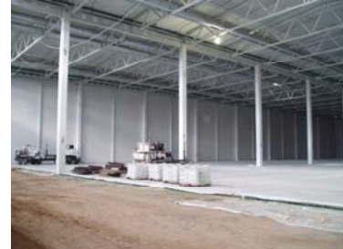
Exterior and interior views of the 16-building, 1,000,000 square meter logistics warehouse complex under construction outside Moscow, Russia, where the Somero SXP Laser Screed is being used to place and finish the concrete floors.
