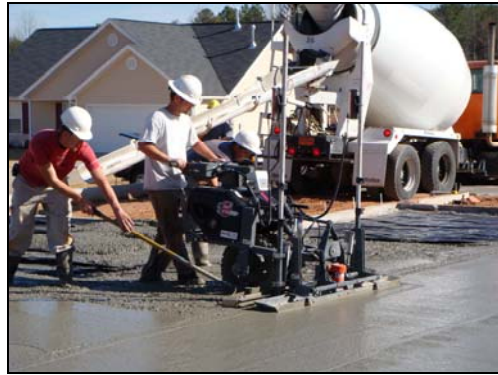
The Somero® Mini Screed™ is ideal for screeding residential and small commercial slabs on grade.
