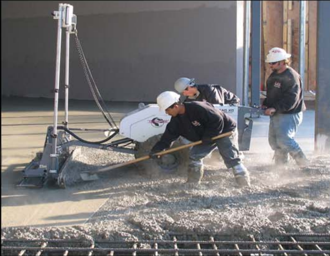
Double Mat Rebar
